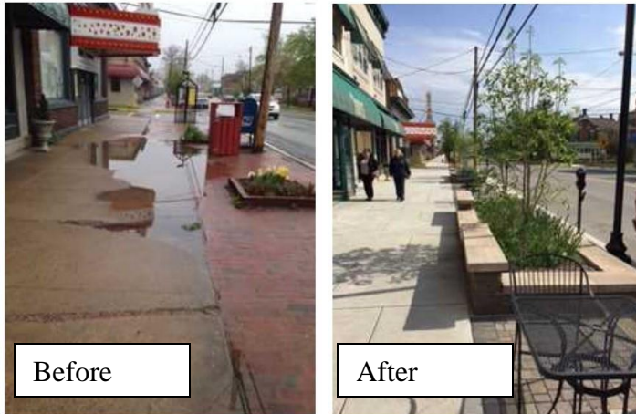
Figure 1: Impact of street tree planter boxes on flooding. Prior to this Chesapeake Bay Trust-funded urban greening grant, local business basements flooded. After the project, businesses report no basement flooding.
