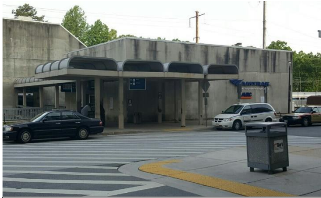
Original BWI Rail Station. Photo by Bob E.
